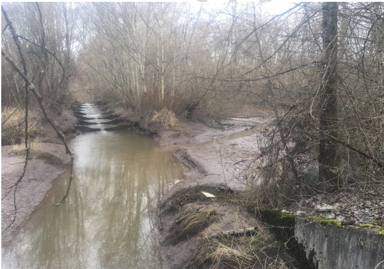
Figure 2: View of the fishway facing west from the access road at the 12-foot-wide concrete bridge crossing. The fishway is clearly visible during a receding tide and acts as the hydraulic elevation control for the wetland. The wetland bottom is currently perched at a higher elevation than the Clear Creek channel by approximately 1 to 3 feet depending on location, and water surface elevation maintained by a
